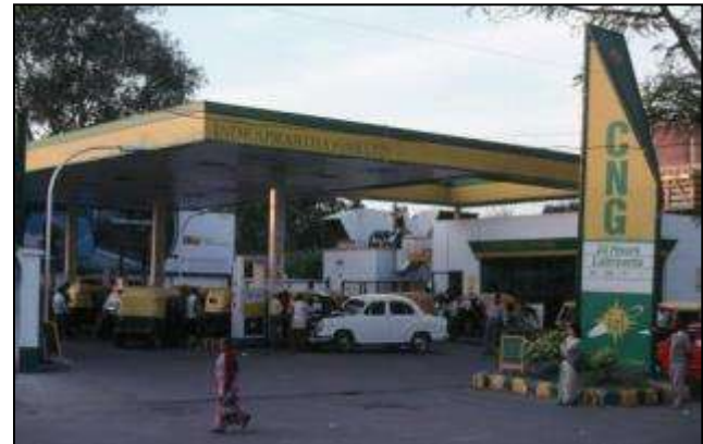
CNG fuel station, Delhi, India
